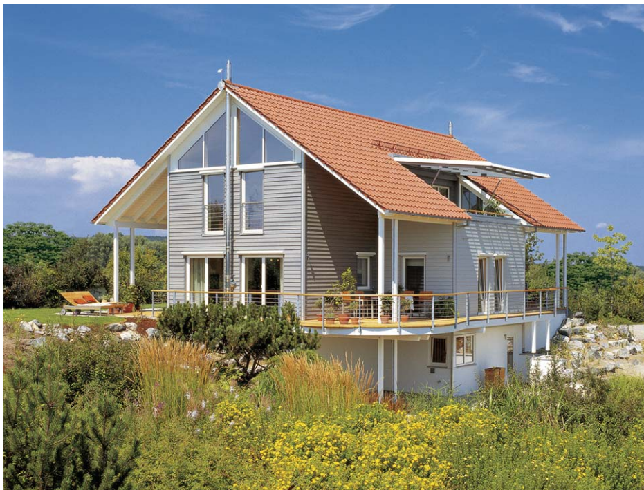
The 108-year-old Baufritz is a firm of architects who are at the forefront of green design for family residences in Germany. Note the greenhouse canopy built into the roof of this Baufritz design.
